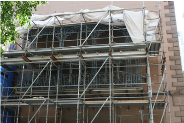
Scaffolding surrounding the East Balcony, July 2012.
